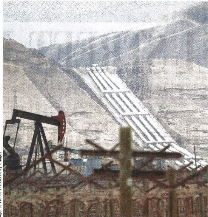
The Chrisman pumps, in the background, are part of the state’s system for redistributing water.
